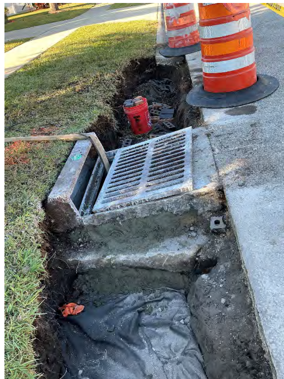
Photo 4661: Underdrain installation right of Inlet 48.
