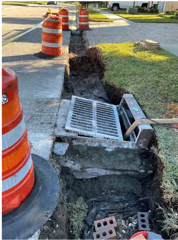
Photo 4660: Underdrain installation left of Inlet 48.
