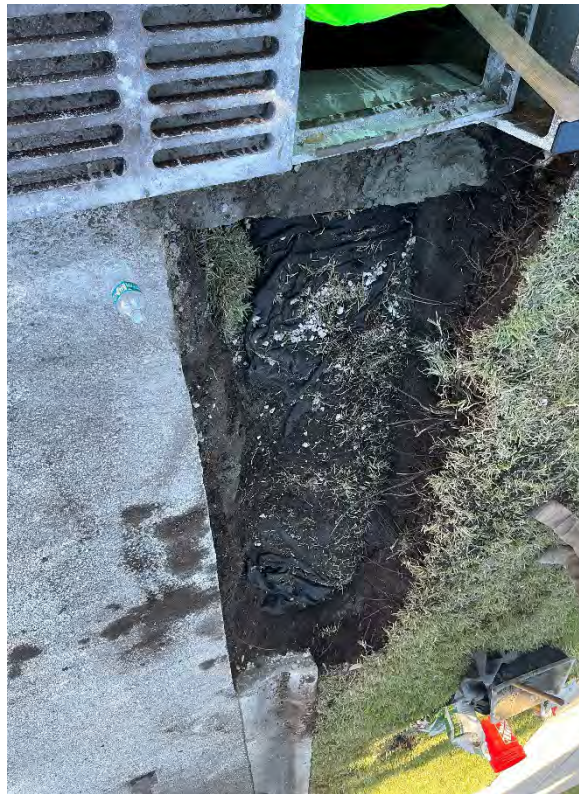
Photo 4650: Underdrain at 2' depth.
