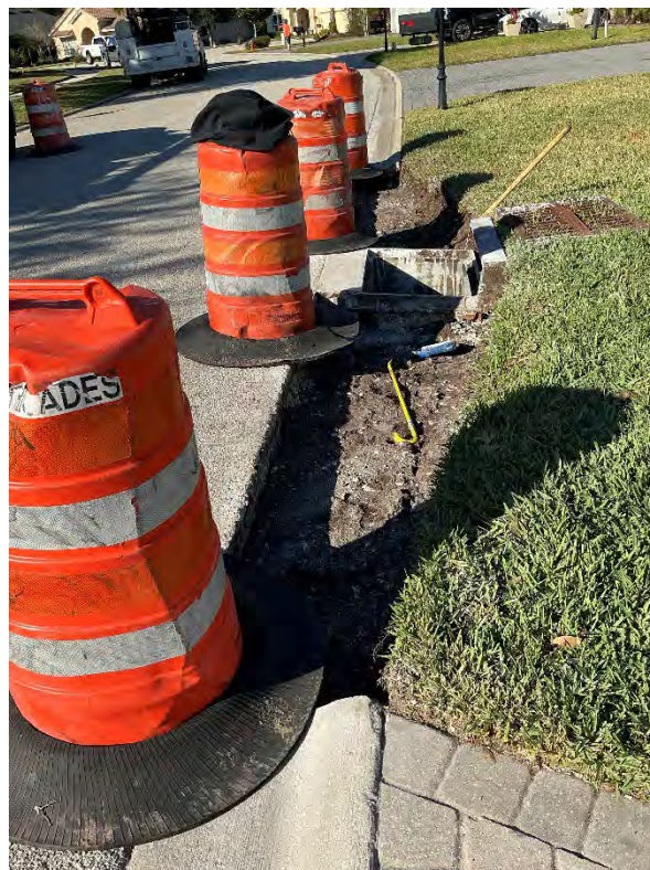
Photo 4652: Removal of existing curb at Inlet 47.
