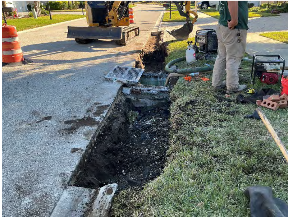
Photo 4647: Removal of existing curb aprons/curb at Inlet 48.
